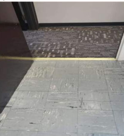
Photo #5 ACM 9" vinyl floor tile and associated black mastic
