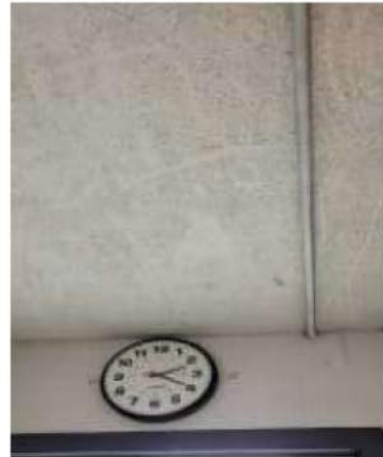
Photo #4 ACM textured plaster ceiling (HA 06)
