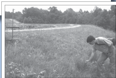
Shown here and above is the Sewanee Utility District's land application system and lagoon (top photo). (Photos courtesy of Dennis George)
