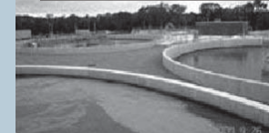
Murfreesboro Wastewater Treatment Plant (Photo courtesy of the City of Murfreesboro)
