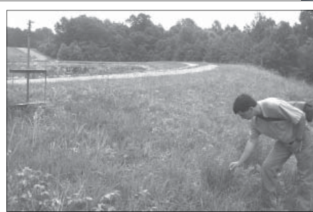
Shown here and above is the Sewanee Utility District's land application system and lagoon (top photo). (Photos courtesy of Dennis George)
