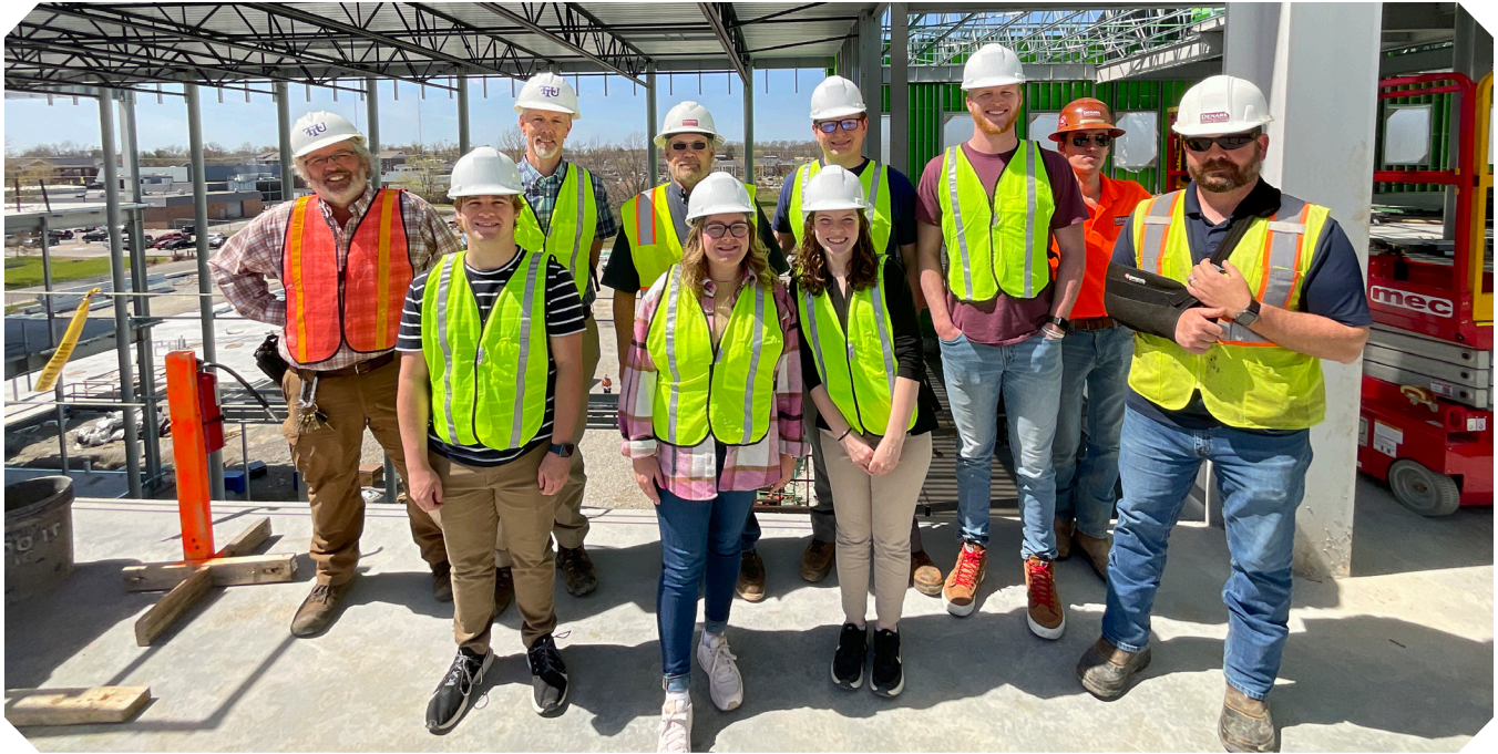
Center for Construction Business Information Modeling staff and students work with Denark Construction and Tennessee Tech construction manager Bill Hall inside the new Ashraf Islam Engineering Building.
