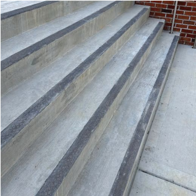
Typical Stair Color: Gray with Light Broom Finish Material: Concrete
