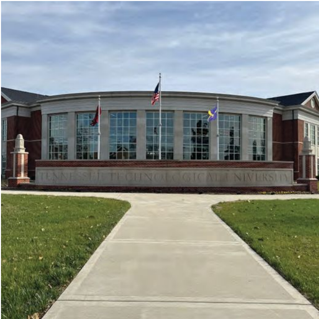
Typical Concrete Walkway Color: Gray Layout: Window Frame with Light Broom Finish
