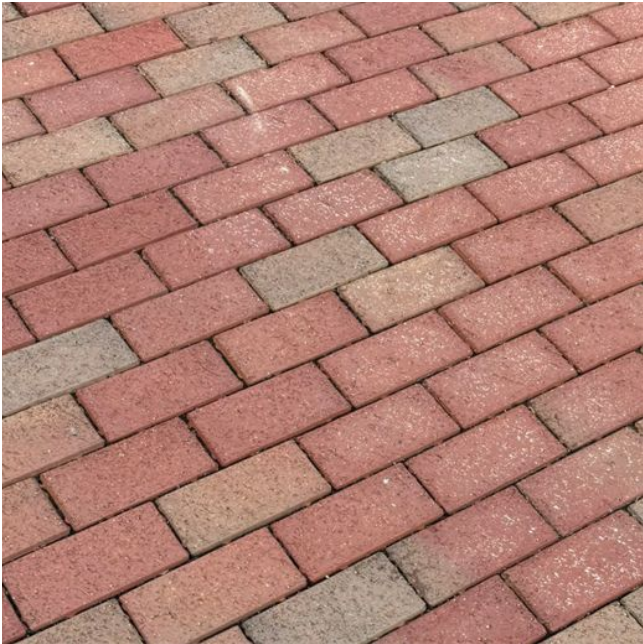
Typical Brick Paving Color: Red Blend Pattern: Running Bond or Herringbone Brick Type: Clay Brick Paving with Beveled Edge
