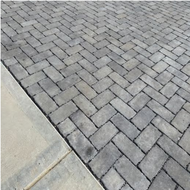
Typical Concrete Pavers Color: Gray Pattern: Herringbone Field
