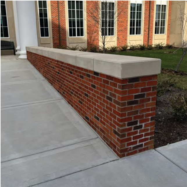
Typical Brick Site Wall Color: Red Brick Blend to Match Campus Architecture Material: Cast Stone Cap with Brick Veneer Base
