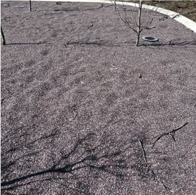
Typical Decomposed Granite Color: Selected by Project Edging: Concrete Border or Metal Edging
