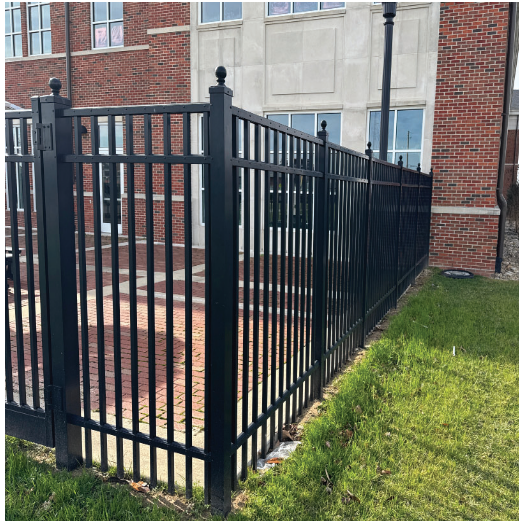
Typical Boundary Fence
