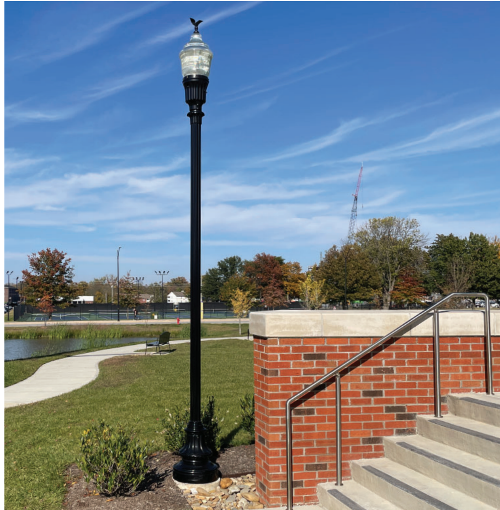
Typical Pedestrian Pole Light
