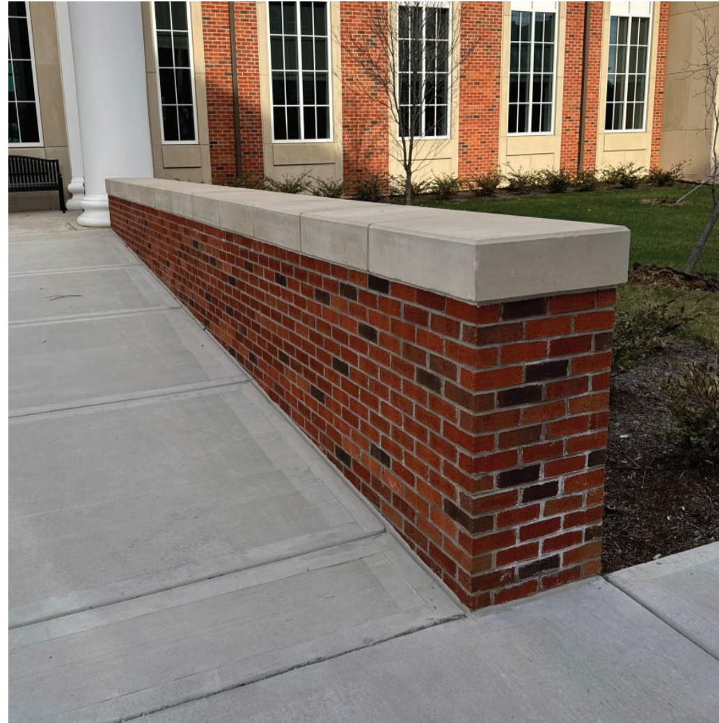
Typical Brick Site Wall
