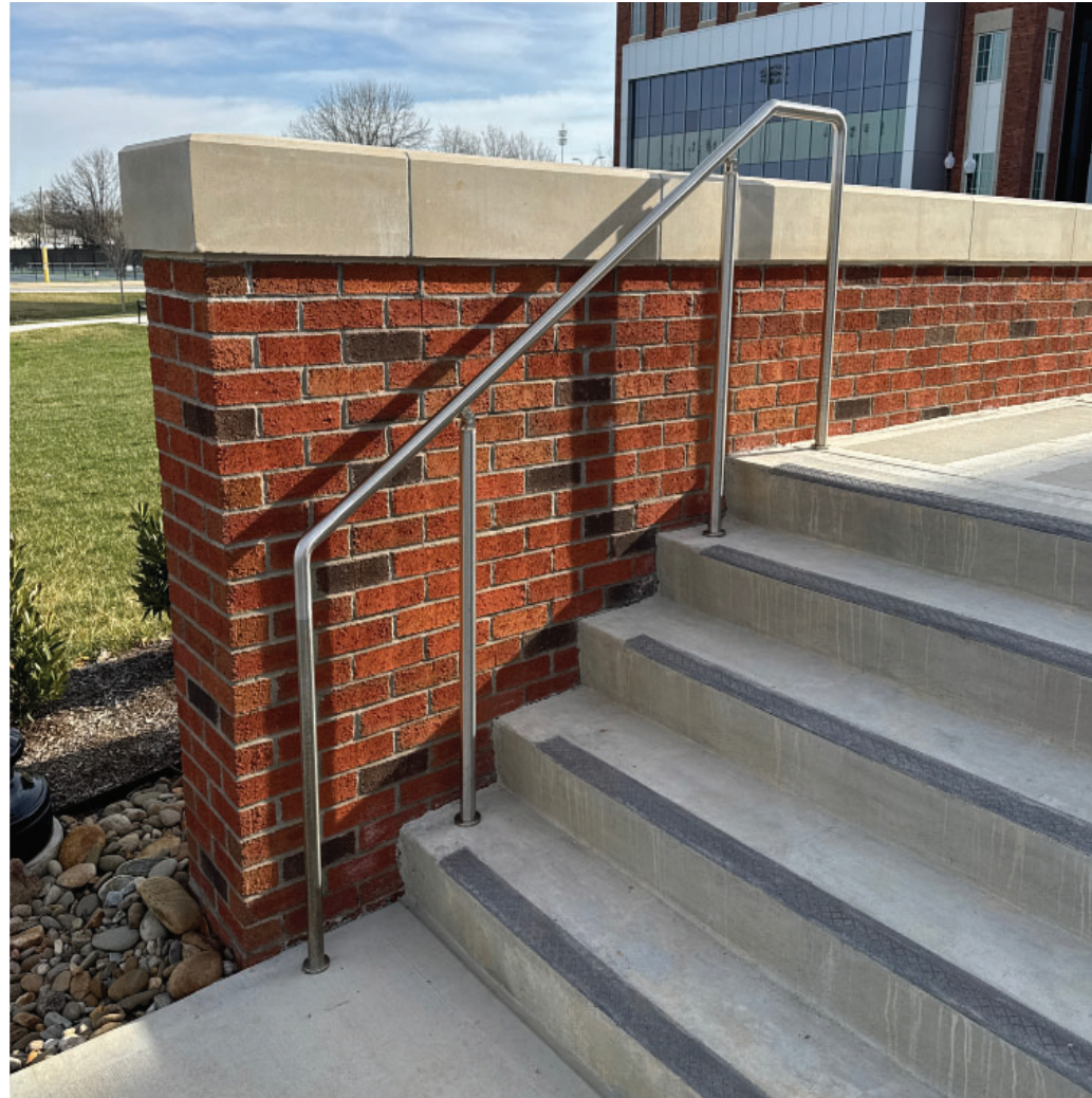
Typical Contemporary Handrail
