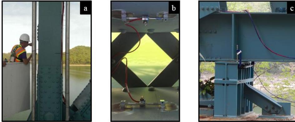
**Figure 10: Installation of Sensing Equipment: a) 2-Inch Strain Gage, b) 6-Inch Strain Gage, and c) Displacement Gage**
