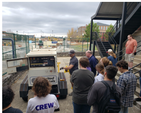
Preparing a large diesel generator for a three phase power feed in preparation for the Children's Concerts.
